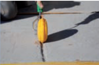
Repaso de juntas con Roler o taco. Going over with roller or block.
